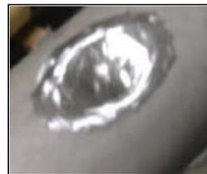
Fig. 3 – Dent ground smooth prior to repair.
