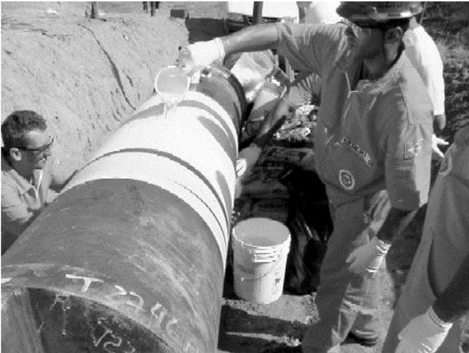
Figure 2 – Field application of a composite repair.
