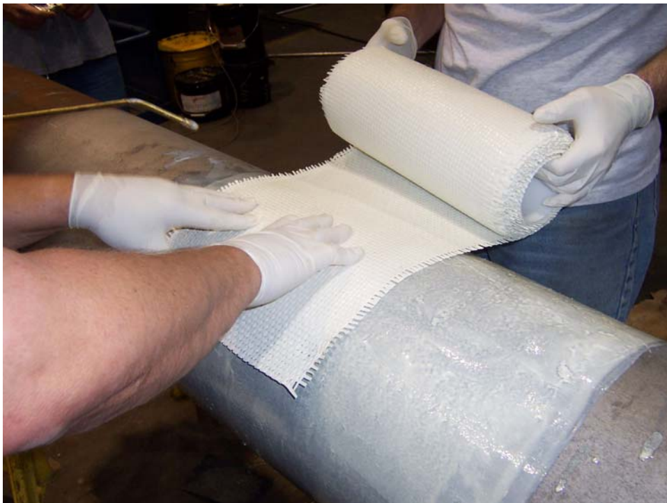
Figure 6 - First layer of Aqua Wrap installed on pipe
