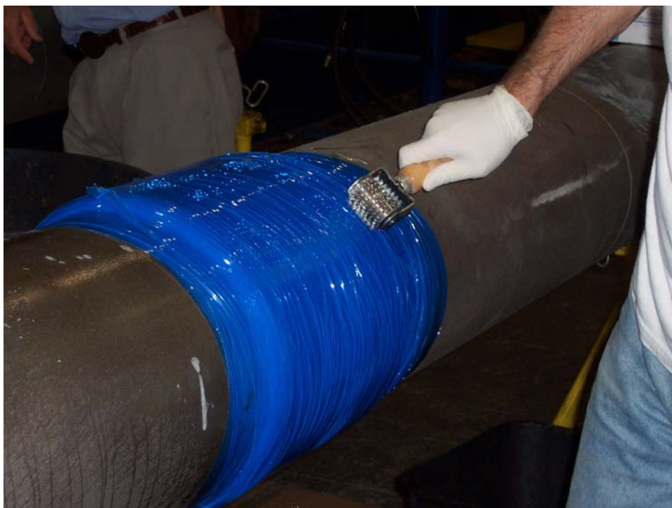
Figure 8 - Perforating plastic wrap to permit off-gassing during cure
