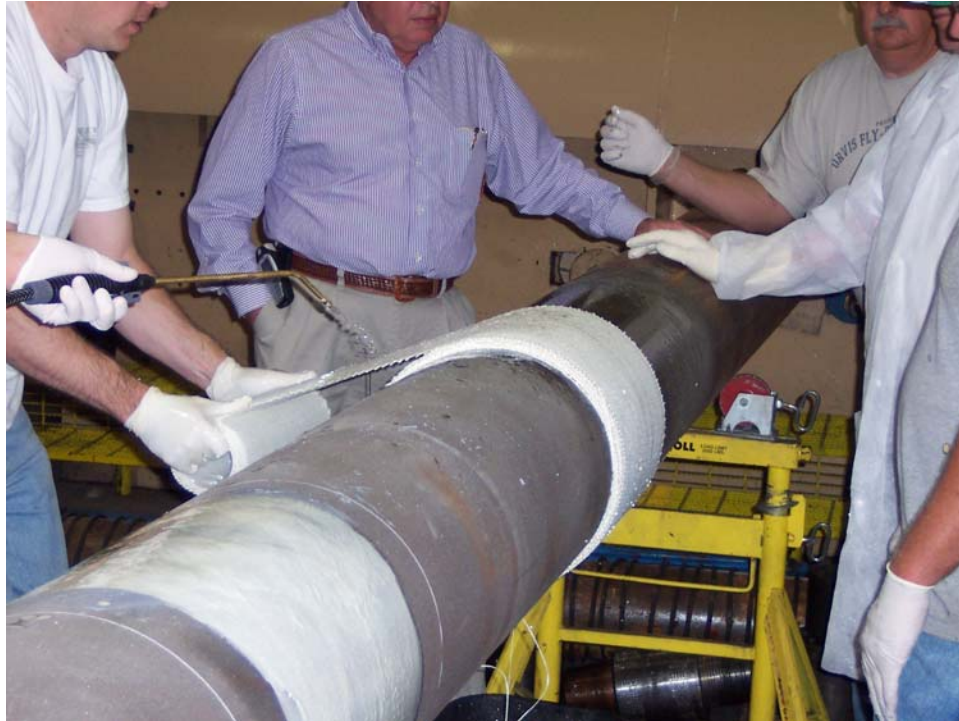
Figure 7 - Continued wrapping of Aqua Wrap in repairing damage
